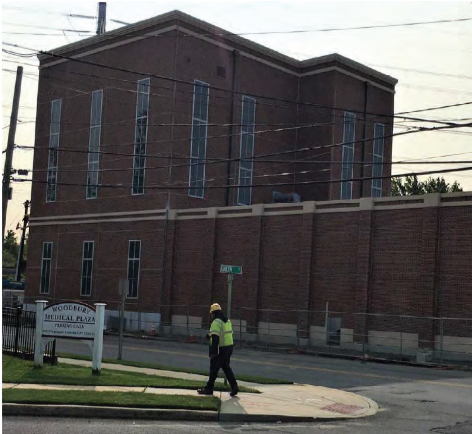
Woodbury Station photo view from Red Bank Ave. & Green St.
