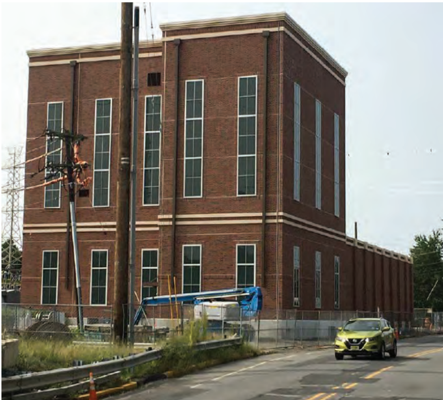
Woodbury Station photo view from below railroad tracks on Red Bank Avenue
